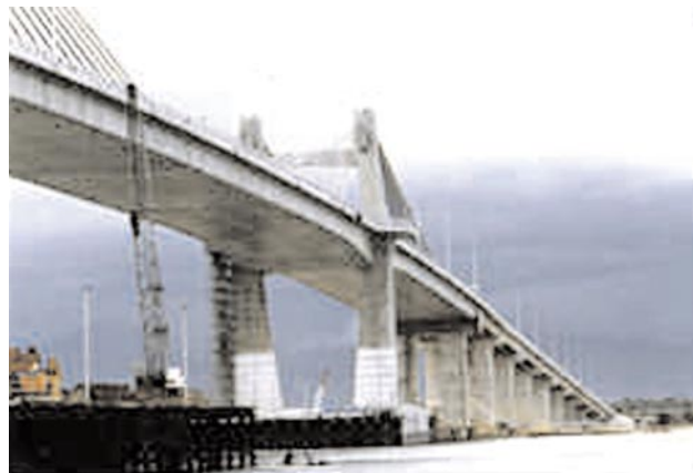
Mandaue-Opon Bridge (Mactan Bridge)
